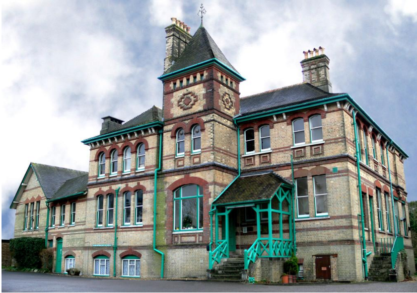
[unfortunately currently covered in scaffolding!]
